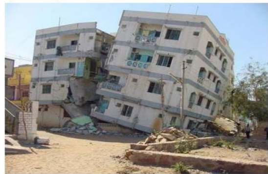
Fig. 2: Building Collapsed in 2001 Bhuj Earthquake
